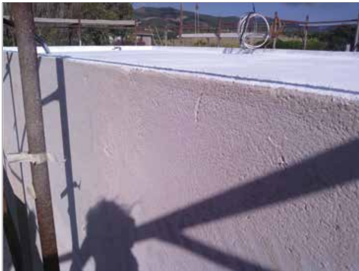
Img 3. North wall surface and roof surface, photographic survey.
