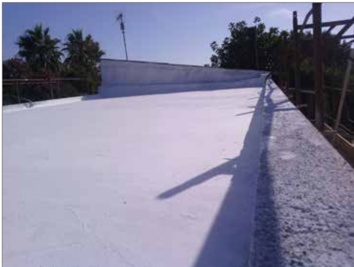
Img 1. Roof surface, photographic survey.
