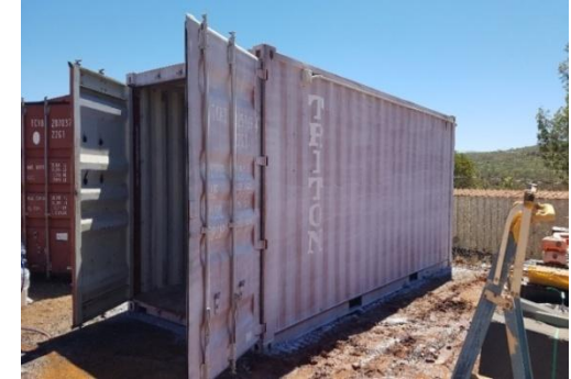
Prime coat complete
