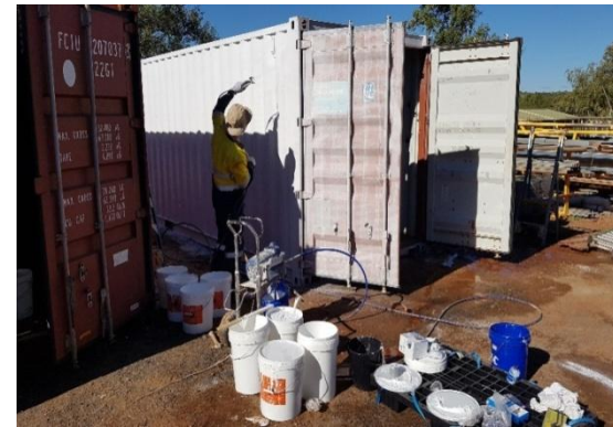
Nearing end of first coat
